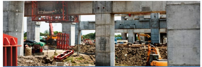
CONSTRUCTION SITE INVENTORY
